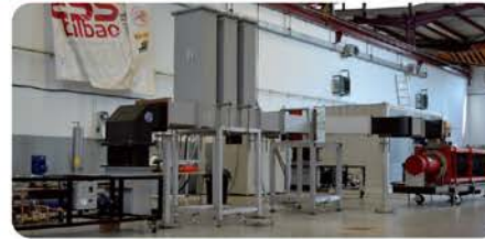
Various RF chains: 1 for the RFQ and 5 for the DTL Composed of modulators, klystrons and wave guides
